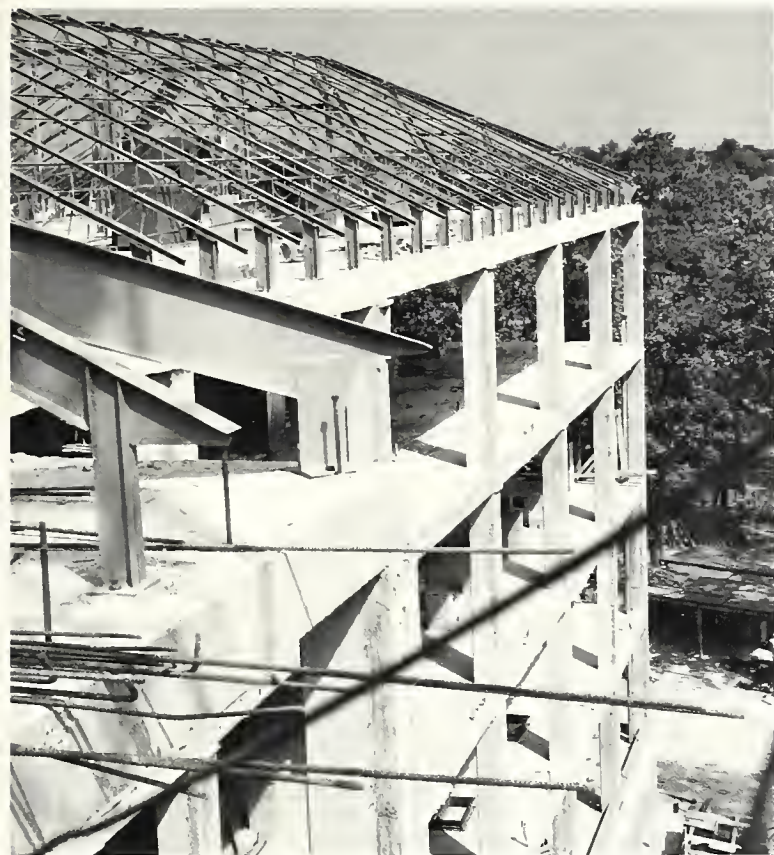
Construction of the new School of Public Health building.
